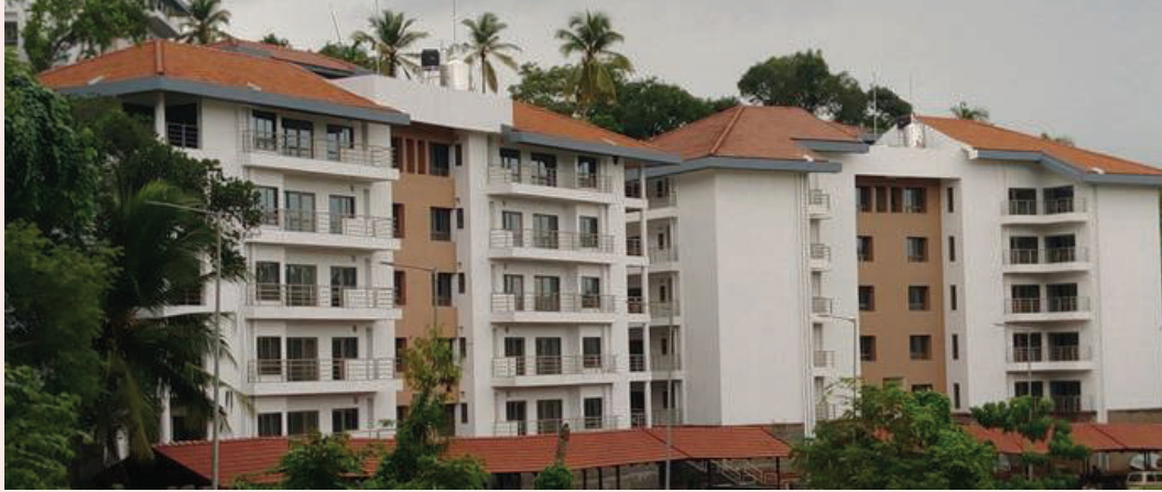
IIMK Phase V (1 st Stage) – Housing Blocks
